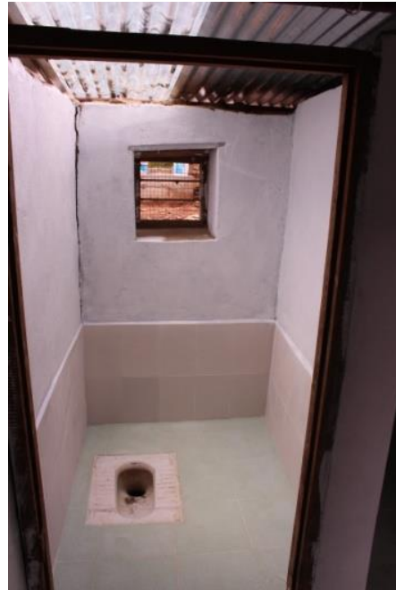
Picture 13 Repair toilet in Indrayani school
