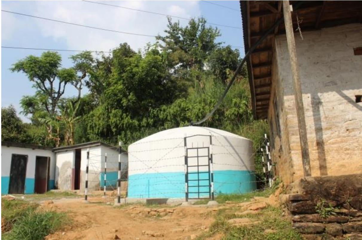
Picture 18 2nd 20-m 3 RWH tank for sanitation facilities in Bishwoshanti School
