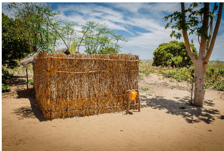
Demonstration of a well-constructed latrine with tip-tap
